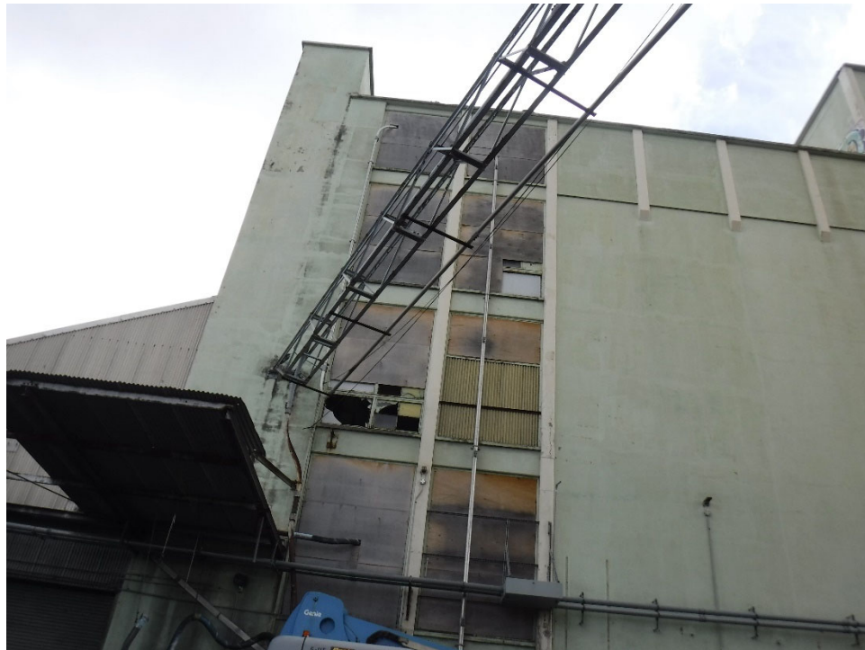
Photo 2: Attachment of lower truss to south warehouse.
