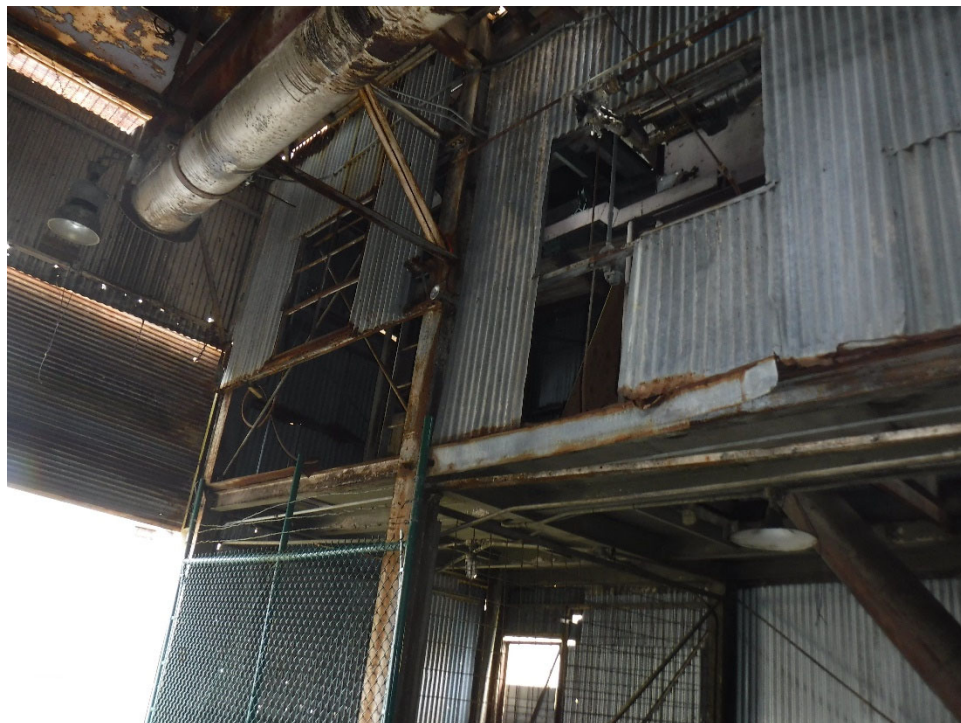
Photo 4: Interior face of attachment of conveyer belt to Husking Shed at north side of silos.
