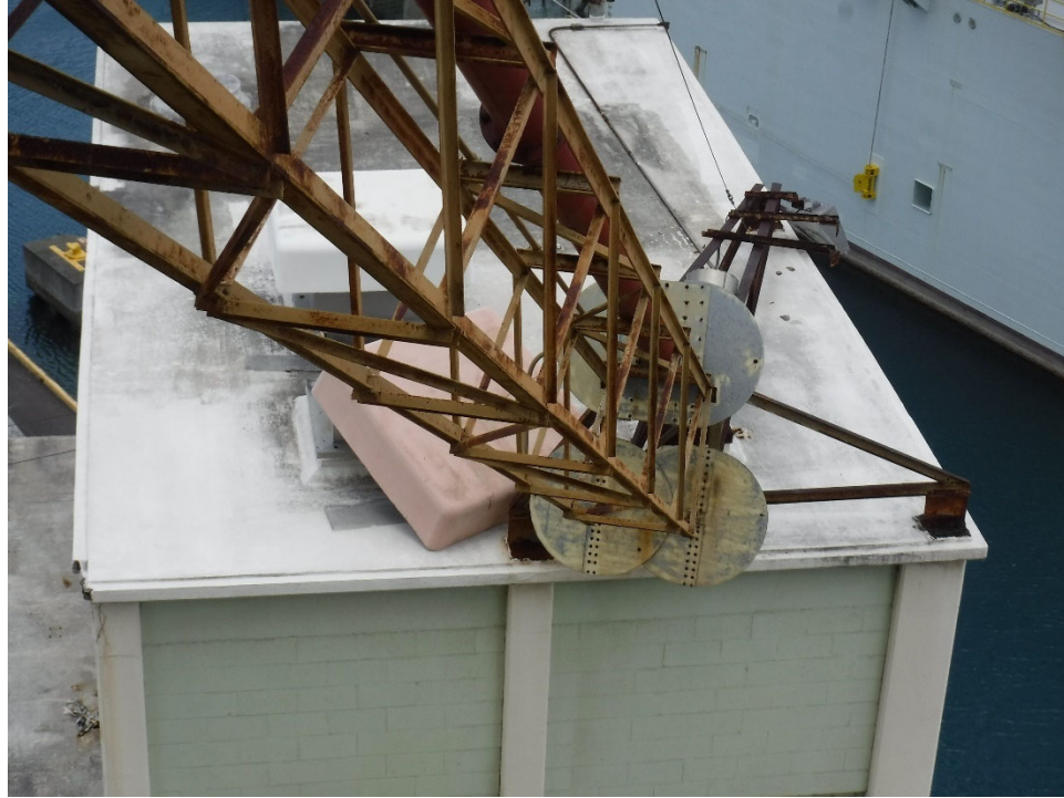
Photo 1: Attachment of upper truss to south warehouse.
